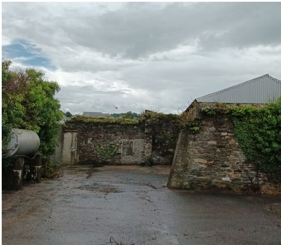
Existing Boundary Wall
